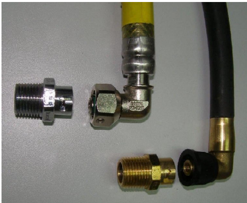
Fig. 2 End connection to the gas installation
