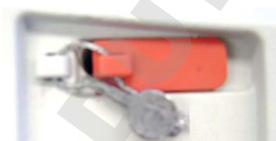
Locked with Wire Seal
